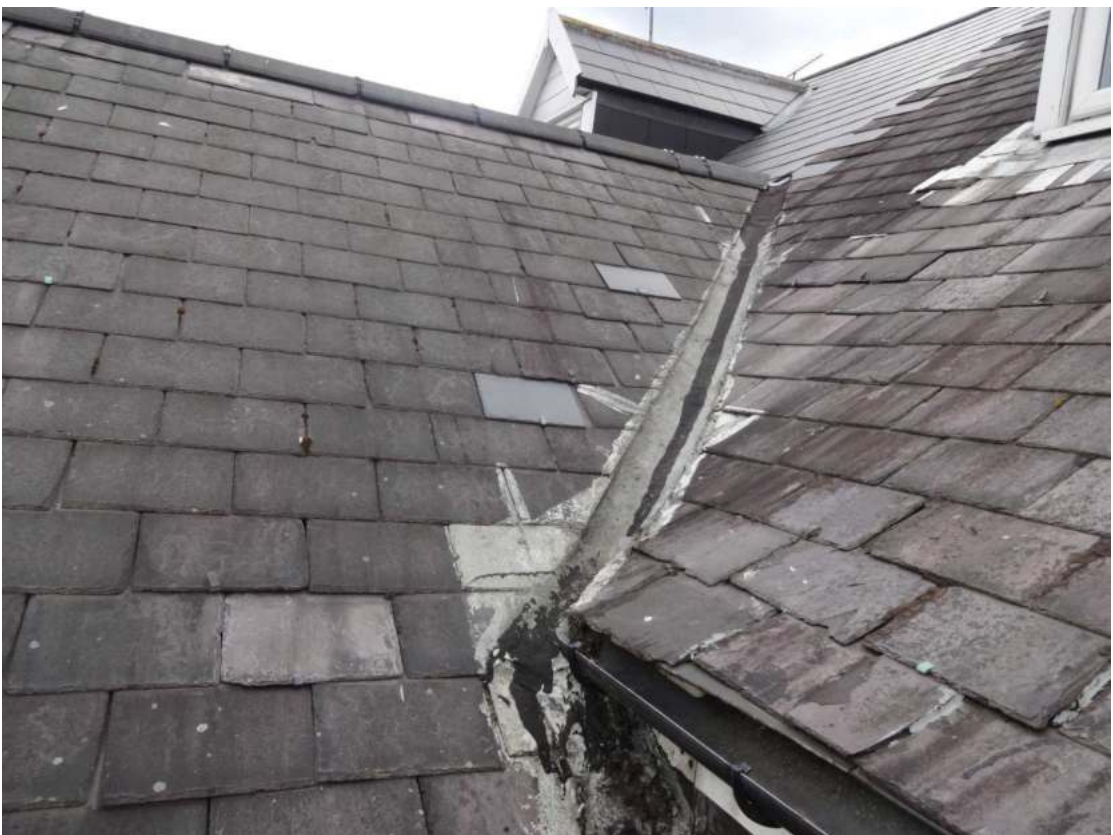
Valley gutter patch painted
