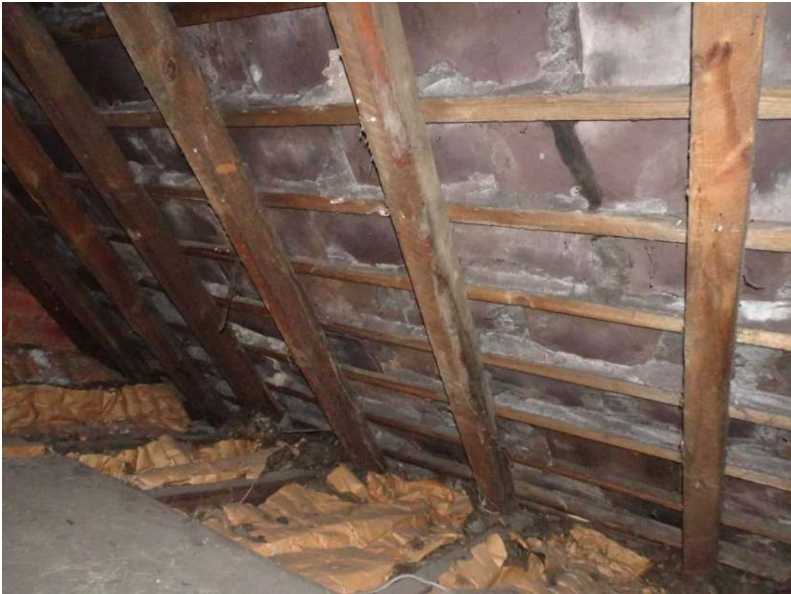
Torching loose to underside of slates
